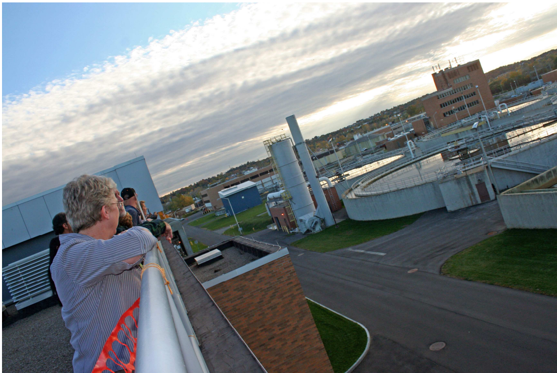
(Metropolitan Waste Water Treatment Facility)
